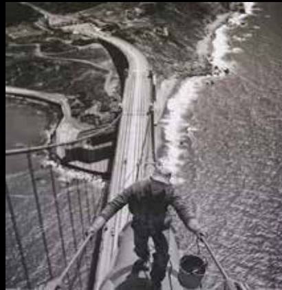
San Francisco: Bridge Maintenance
