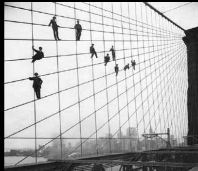
New York: Bridge Maintenance
